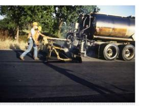
Needle-punched fabric is thicker, fuzzy, softer and more pliable making it ideal for the paving application. They install smoother with fewer wrinkles due to their high elongation (stretch). Numerous reports state the fuzzy side placed into the asphalt oil provides reinforcement at the interface. The fuzzy side provides a greater effective surface area of the fabric, offering better adhesive and shear strength with less slippage.
