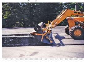
Often manufacturers roll their material for machine placement, so the fabric comes off the roll and goes underneath the roll rather than coming off the top and this places the heat bonded side up and fuzzy side down. The roll must be loaded correctly onto the machine.
