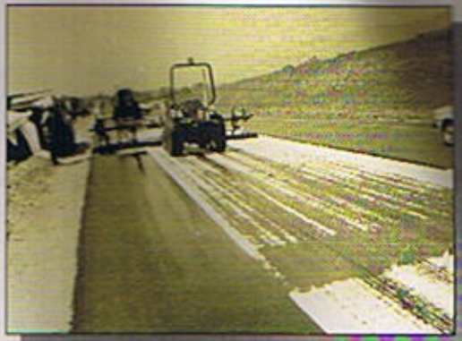
Thin fabric doesn't hold tack coat as easily, resulting in bleed through, which can be hazardous to workers and equipment.
