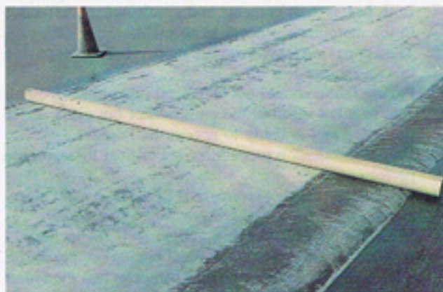
Figure 4: Roll core shows amount of fabric shrinkage observed in Los Angeles County.
