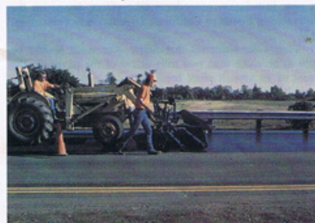
Figure 2: Fabric installation equipment has been mounted on tractors, fork lifts and skid loaders.
