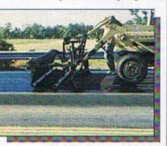
Some machines have features that can place fabric next to guard rails, curbs, prior asphalt passes and walls.
