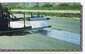
In some states such as Illinois 2- and 3-ft, fabric is used to cover edge drain trenches.
