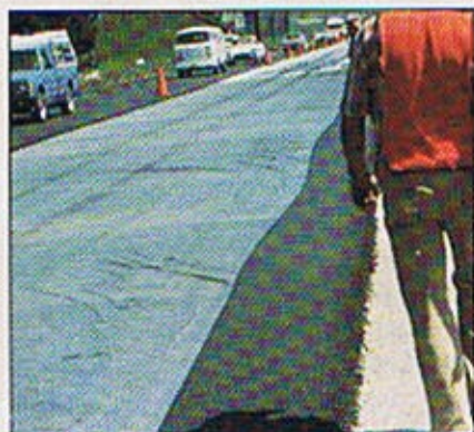
When dual heat-bonded fabric is changed to fabric heat-bonded only on one side, bleed-through stops because the fabric is more absorptive.
